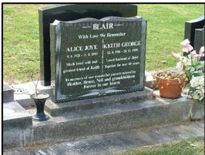
Book shaped (T28) grey plate on a standard two-step plastered concrete base.
