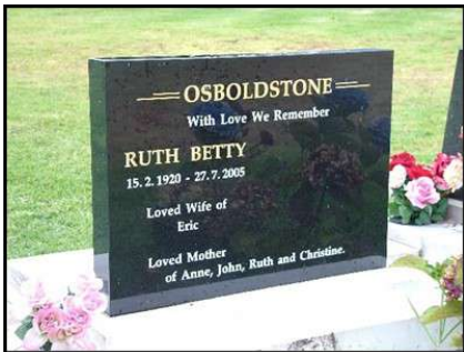
Rectangular plate headstone (75mm) on a standard two-step plastered concrete base.
